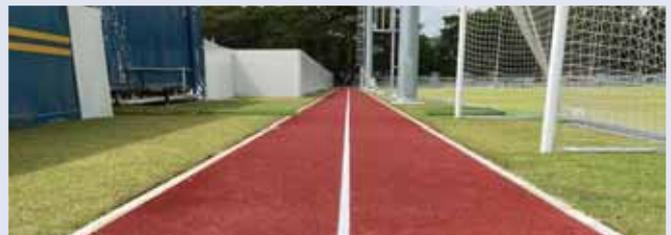
(Top) Process behind repurposing the old shoes and (Bottom) 108m running track built using recycled rubbers granules
